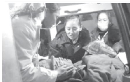
A worker receives medical treatment after being carried out from a collapsed highway tunnel in the Degan Tibetan Autonomous Prefecture in southwest China's Yunnan Province, on 12 Aug, 2011. All eight workers trapped in the collapsed tunnel on Thursday have been saved and sent to hospital for treatment by 11:50 pm Friday. The workers currently were in normal condition, according to local authorities.—XINHUA
