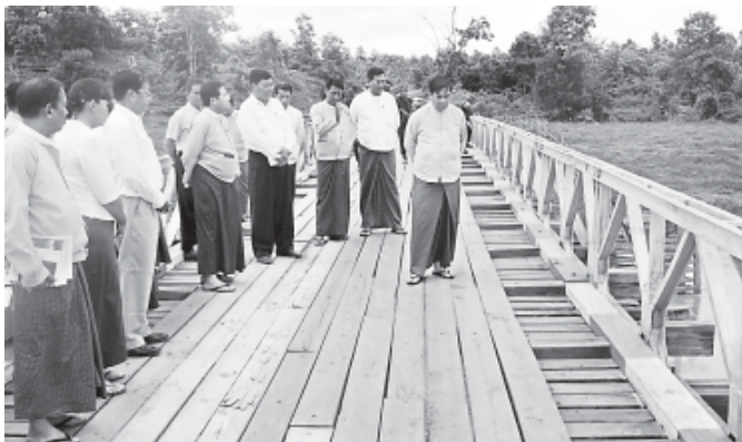
Chief Minister of Sagaing Region U Tha Aye inspects maintenance of bridge across Namma Creek. —MNA
