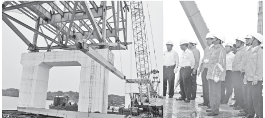
Union Minister U Khin Maung Myint inspects Ayeyawady Bridge (Nyaungdon).—MMA
