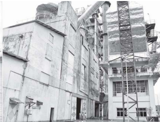
Vice-President Thiha Thura U Tin Aung Myint Oo visits No. 1 Cement Plant (900 tons) in Hpa-an Township.—MNA
