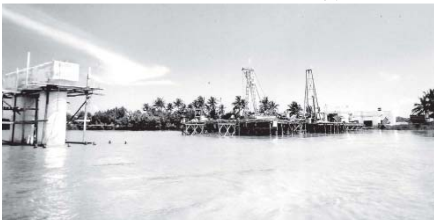
Hlinephone Bridge Project is due to be completed ahead of schedule.
