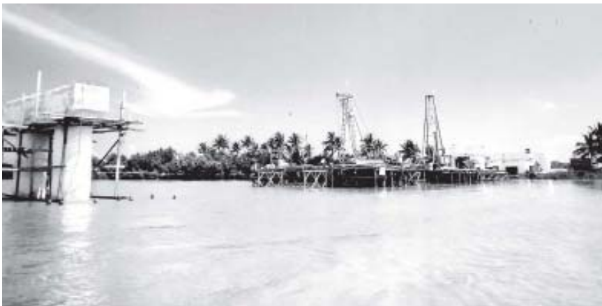
Hlinephone Bridge Project being implemented across Hlinephone Creek in Mawlamyinegyun Township.
