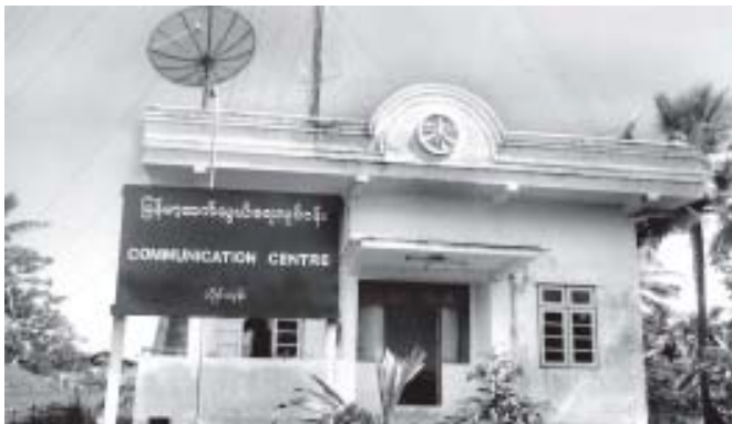
Photo shows communication centre of Myanmar Posts and Telecommunications.
