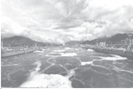
Photo taken on 14 July, 2011, shows a corner of the first sewage treatment plant in Lhasa, capital of southwest China's Tibet Autonomous Region. The first sewage treatment plant in Lhasa was completed and put into test operation on Thursday. The plant adopts CAST biological treatment and has a daily sewage treatment capacity of 50,000 tons. Funded by the central government, the total investment of the plant is 122 million Yuan.—XINHUA
