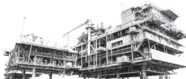
Photo taken on 13 July, 2011 shows Suizhong 36-1 oilfield on Bohai Sea, offshore the northeast China's Liaoning Province.—XINHUA
