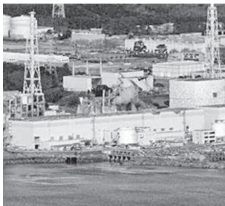
An aerial view shows Fukushima Daiichi nuclear power plant in Fukushima.
