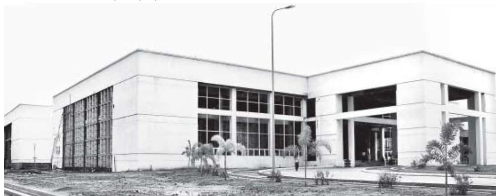
Photo shows progress of National Museum (Nay Pyi Taw).—MNA
