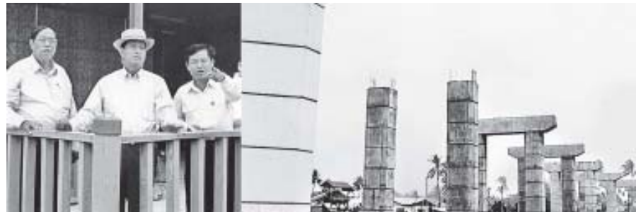
Union Minister for Construction U Khin Maung Myint inspects construction of Bogale River-crossing Bridge.—MNA
