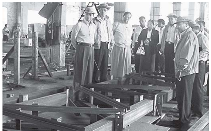
Union Minister for Construction U Khin Maung Myint inspects preparation for major repair of Jiang (Kawkareik) bridge.—MNA
