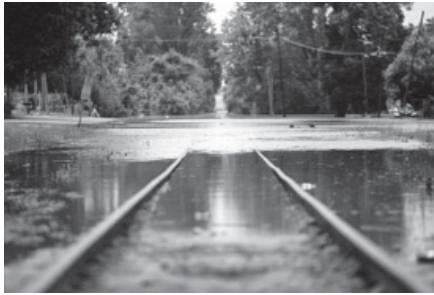
Flooded railroad tracks run near the Mississippi River in Vicksburg, Mississippi. Historic flooding along the Mississippi River turned deadly Thursday when an elderly man died despite being pulled from floodwaters and resuscitated by firefighters.—INTERNET
