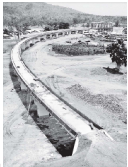
The approach railroad to Ayeyawady Bridge (Sinkhan).
