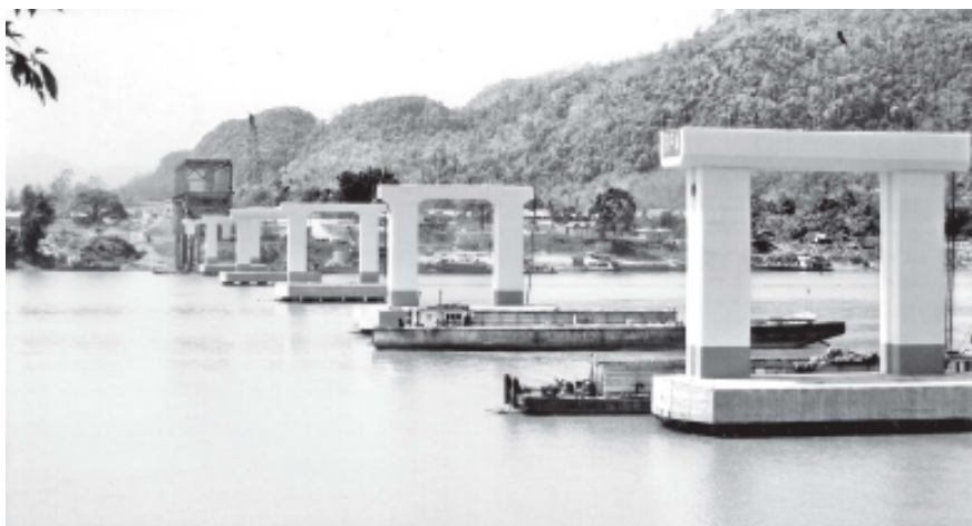
Piers for Ayeyawady Bridge (Sinkhan).
