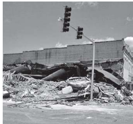
A building that housed a beauty parlor in downtown Morrilton, Ark collapsed Monday, 16 May, 2011, killing a young girl and injuring at least five other people. According to police, rescue teams are searching the wreckage for possible survivors but they think most people escaped. INTERNET
