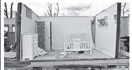
A room is exposed in a destroyed house in the devastated town of Pleasant Grove, Alabama, on 1 May.—INTERNET
