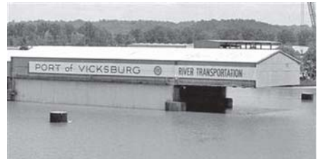
Backwater from the swelling Mississippi River engulfs a storage facility at the Port of Vicksburg in Vicksburg, Mississippi 13 May, 2011.—INTERNET
