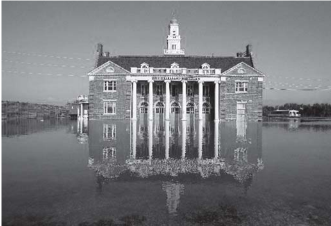
Water from the swollen Mississippi River surrounds the Historic Yazoo & Mississippi Valley Railroad Company Depot in Vicksburg, Mississippi on 10 May, 2011. More residents were warned on Monday to get out of the way of the raging Mississippi River as it surged toward a near-record crest in its southern reaches, prompting authorities to try to divert some of the flood waters.—XINHUA
