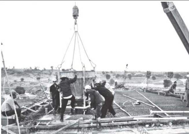
Workers building Ayeyawady Bridge (Malun).
