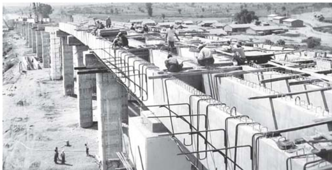
Photo shows approach bridge of Ayeyawady Bridge (Malun) on Malun bank.
