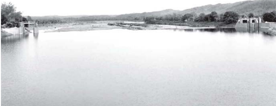
IRRIGATION FACILITY IN MAGWAY REGION: Aingma Diversion Weir was built on Mann Creek near Aingma Village of Minbu Township, Minbu District, Magway Region in 1891. The 580 feet long and 10 feet high concrete facility is supplying water to annual and perennial crops on irrigated areas.
