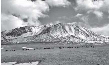
Photo taken on 2 May, 2011 shows the plateau landscape beside the Xinzang Road in construction in Ritu County of Tibet Autonomous Region. Xinzang Road is a plateau road connecting northwest China's Xingjiang Uygur Autonomous Region and southwest China's Tibet Autonomous Region. The workers currently are building the highest part of the road, with an average altitude of 5,000 metres, in the condition of oxygen deficit and cold weather.
