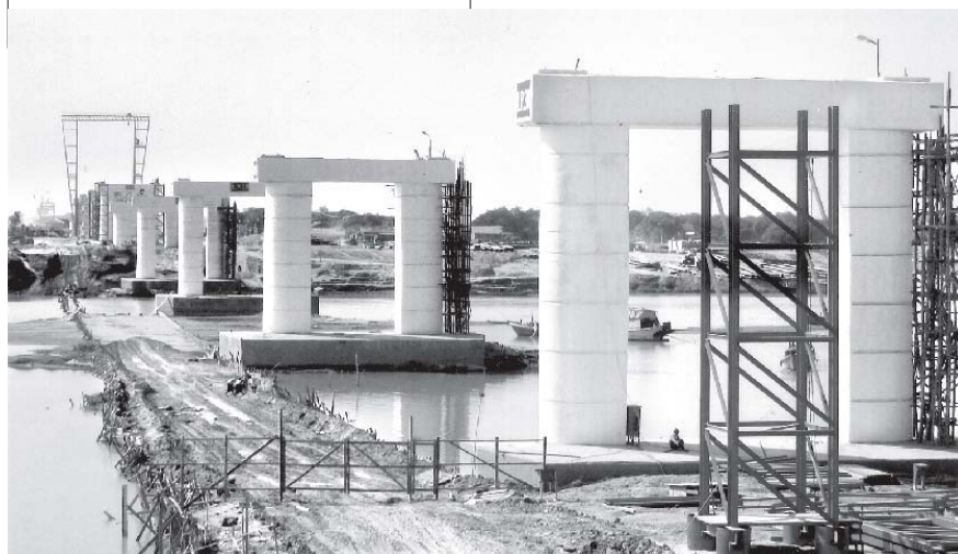
Ayeyawady Bridge is under construction with piers.
