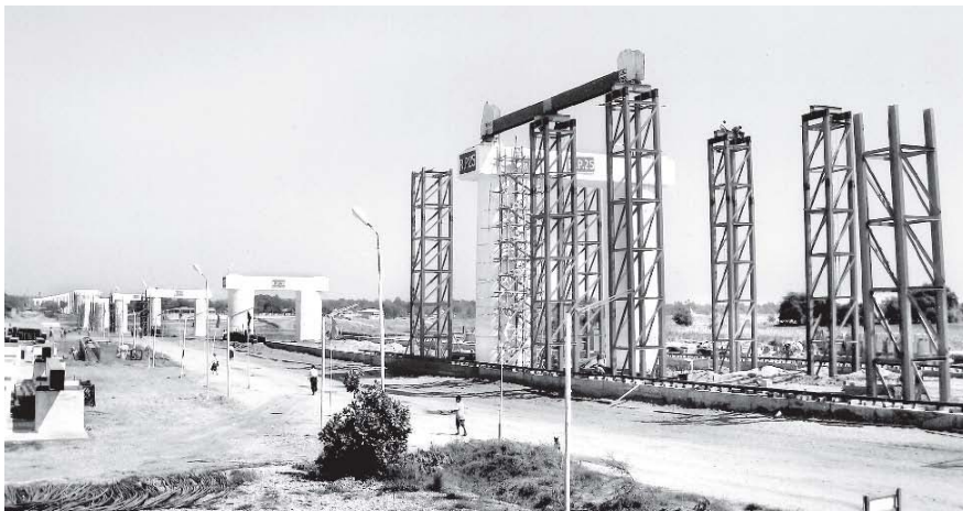
Photo shows installation of steel frames for the bridge on Pakokku bank.
