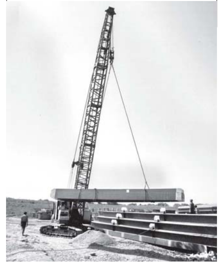
A crane lifting steel frame imported from China DAMC Engineering Co Ltd.
