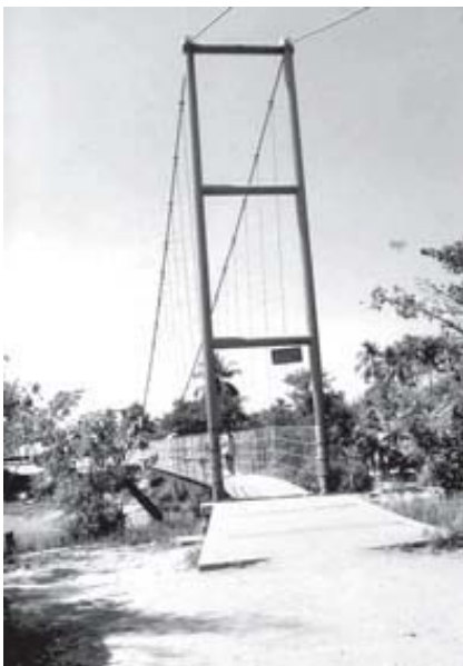
The suspension bridge crossing Bago River.
