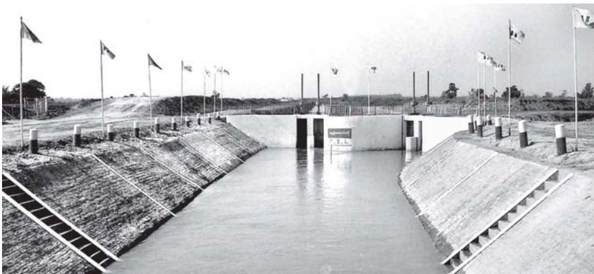
Ayethaya Diversion Weir and diversion structure benefitting farmlands.
