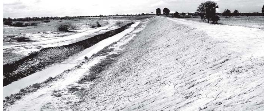
The 3500 feet long and 10 feet high embankment of Letse Dam near Ywathikalay Village, Yagyi Village-tract, Pyawbwe Township.
