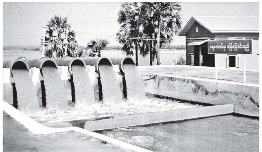
Ngathayouk River Water Pumping Station, one of facilities for improving of agricultural sector.
