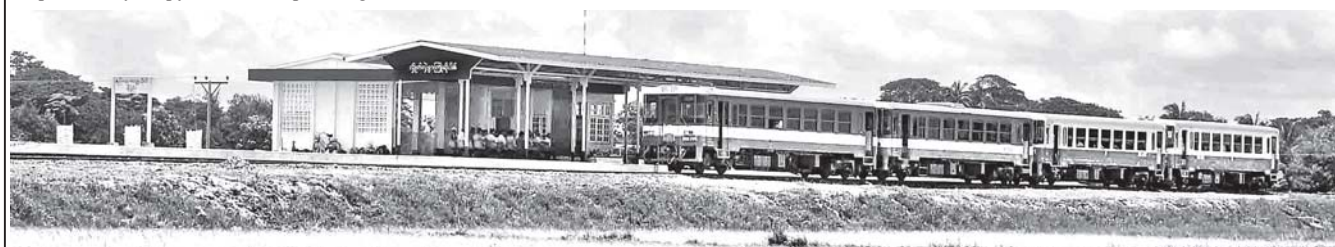
Pyay (Shwedaga)-Paukkaung railroad section commissioned as a railroad network across the nation.
