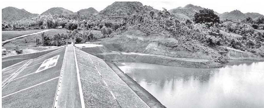
Nantkyan reservoir seen for supply of irrigation and drinking water.
