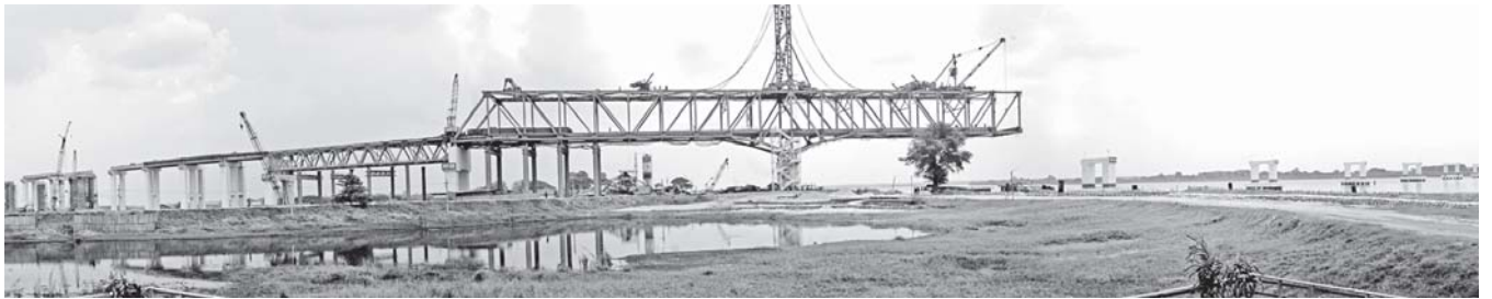
Construction of Ayeyawady Bridge (Nyaungdon) in progress.—MNA
