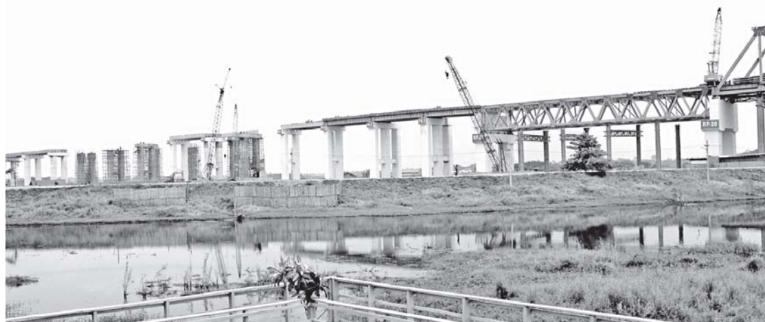
Progress in construction of Ayeyawady Bridge (Pakokku).—MNA
