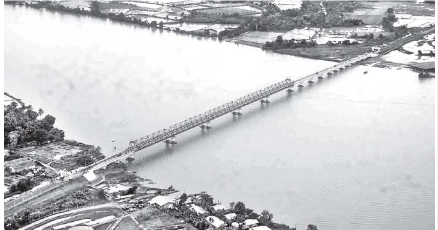
Aerial view of Yazudaing Bridge No. 1 in Ayeyawady Region.
