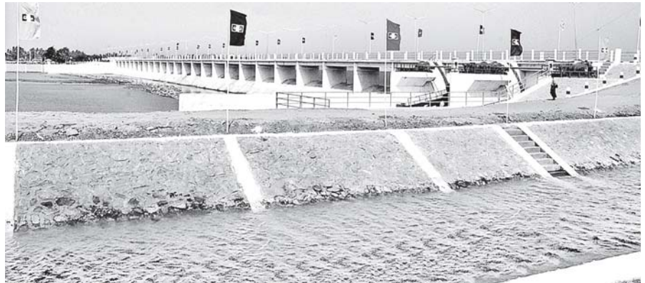
Photo shows Paunglaung Diversion Wier in Nay Pyi Taw Pyinmana Township.
