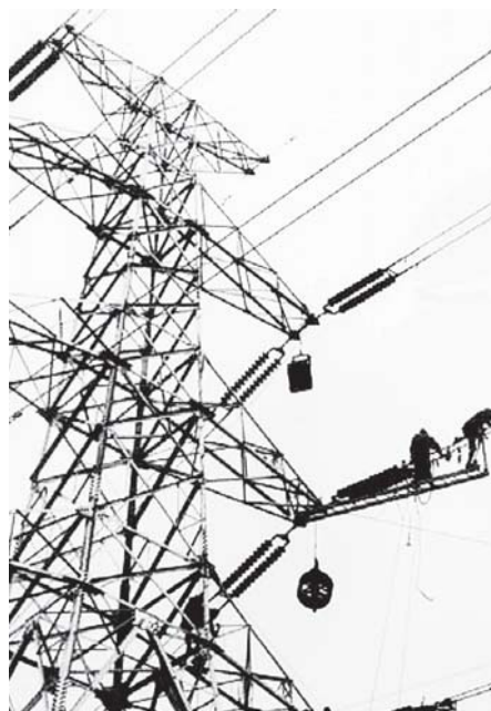
Photo Shows Shweli-Mansan-Shwesayan 230-KV Power Grid Project.
