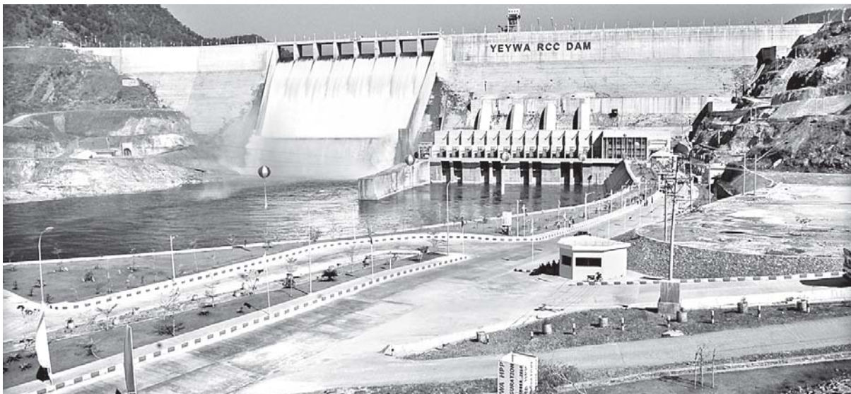
Yeywa Hydropower Project that can generate 3550 million kwh a year seen near Yeyaman Village, 31 miles southeast of Mandalay.
