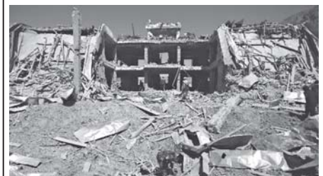
An Afghan investigator inspects at the place of suicide car bomber in front of the district administrative building in Musayi district, south of Kabul, Afghanistan, on 14 April, 2011. XINHUA
