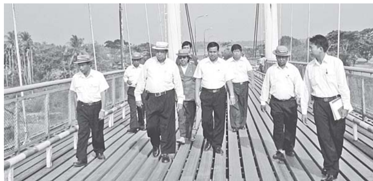
Deputy Construction Minister U Soe Tint walks along Myingka-seik suspension bridge.
