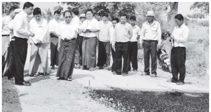
Ayeyawady Region Chief Minister U Thein Aung inspects maintenance of Maubin-Hsamalauk road.—MNA
