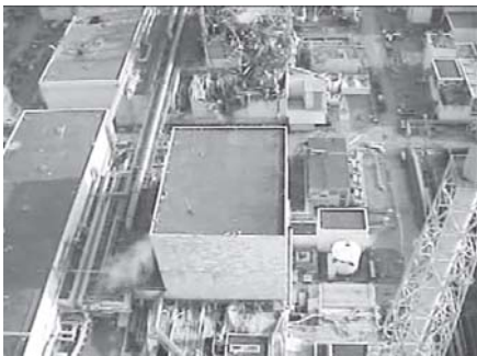
This Sunday, 10 April image taken by T-Hawk drone aircraft and released by Tokyo Electric Power Co (TEPCO) shows the reactor building of Unit 2, centre, of the tsunami-crippled Fukushima Dai-ichi nuclear power plant in Okuma town, Japan nuclear agency announced on Tuesday that it has raised the severity level of the accident at the crippled Fukushima No1 nuclear power plant to 7, the worst on an international scale, from the current 5.
