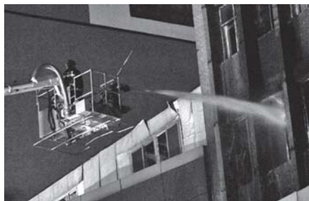
The fire occurred in a large shopping mall has been put out in Xining, capital of northwest China’s Qinghai Province, on 10 April, 2011. After over 10 hours’ efforts, the fire has been extinguished at 1:49 am Sunday. The fire has caused a cleaner of the shopping mall dead and 15 people wounded as of the press time. INTERNET
