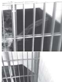
The photo from Tokyo Electric Power shows radioactive contaminated water from the crippled Fukushima Daiichi Nuclear Power Plant No 2 reactor, leaks through a crack in a concrete pit and drains into the ocean in Fukushima prefecture, northern Japan 2 April, 2011 (Top) and the water leak halts on 6 April, 2011 (Bottom).
