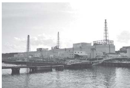
This picture taken by Japan's Maritime Self Defence Force, shows the badly damaged Tokyo Electric Power Co (TEPCO) No 1 Daiichi nuclear plant at Okuma town in Fukushima prefecture.—INTERNET
