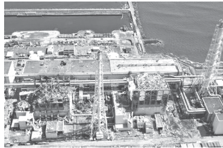
In this 24 March, 2011 aerial photo taken by a small unmanned drone and released by Air Photo Service, damaged Unit 3, left, and Unit 4 of the crippled. INTERNET
