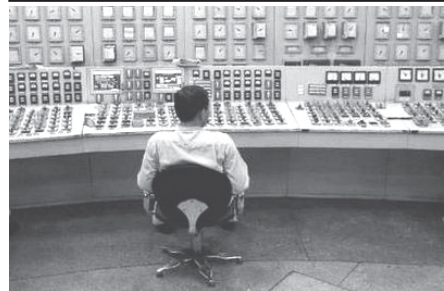
A worker sits at a control table in the operation centre of the Pha Lai Thermal Power Plant, 70 km (43 miles) northeast of Hanoi, on 24 March, 2011. The coal-fired plant's first generator began operations in 1983 and now, the plant's six generators provide about 8 percent of Vietnam's energy needs.—INTERNET
