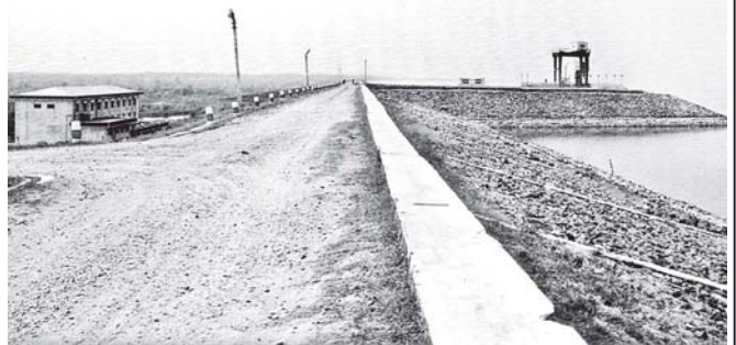
The hydropower plant of Thaphanseik Dam in Sagaing Region.
