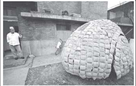
The egg house more than 2m high, 3m long and 2m wide. Its outside wall is made of bamboo splints and gunnysacks which filled with sawdust and grass seeds for keeping warm.
