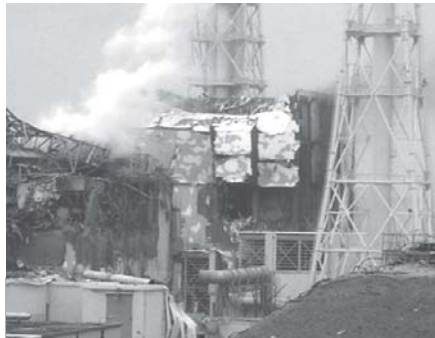
The photo released by Tokyo Electric Power Co on 16 March, 2011, shows No3 reactor (L) and No4 reactor of the Fukushima Daiichi plant. The fire struck on early Wednesday at the building housing of the No4 reactor of the Fukushima Daiichi plant, 240 km (150 miles) north of Tokyo.
