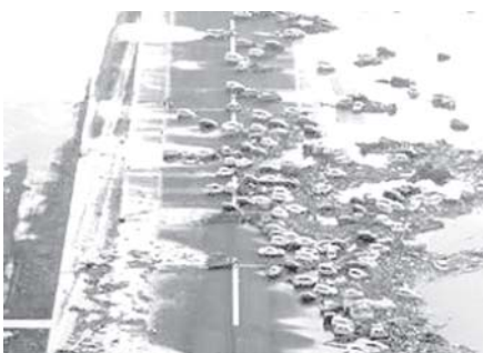
Cars and debris litter a runway at Sendai Airport in northern Japan.— INTERNET
