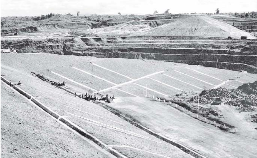
A dike under construction in Kanyin Dam Project.
