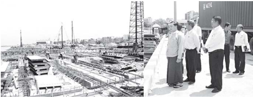
Minister for Transport U Thein Swe inspects construction of jetty at Asia World Port.—MNA
