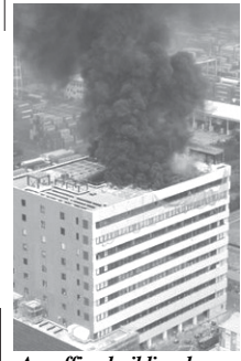
An office building burns in Tokyo after an earthquake on 11 March, 2011.—INTERNET
