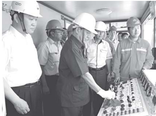
Minister for Energy U Lun Thi starts drilling riverbed with the use of Horizontal Directional Drilling Machine for Ayeyawady River Crossing Pipeline.
