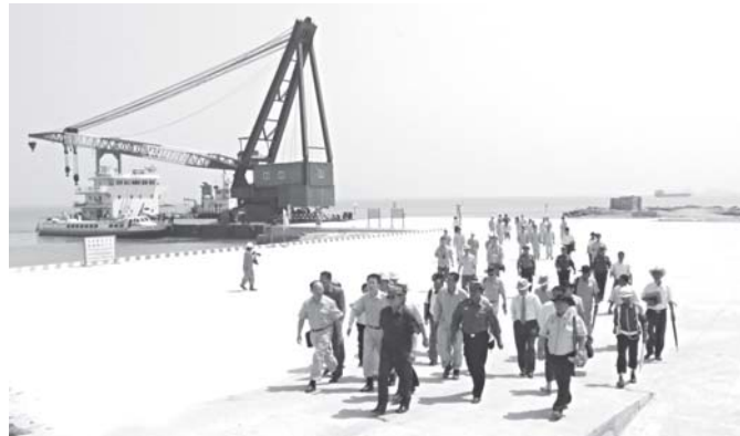
Minister for Energy U Lun Thi at the construction site of Myanmar-China crude oil pipeline project in Made Island, Kyaukpyu Township.—MNA
