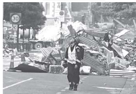
A rescue worker walks through the rubble in central Christchurch 2 March, 2011.
