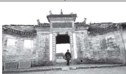
Photo taken on 3 March, 2011 shows the front gate of the Hakka Dongsheng enclosed house in Anyuan County, east China’s Jiangxi Province. Dongsheng house, one type of the typical Hakka dwellings with 94 metres long and 73 metres wide, is the largest square enclosed house for Hakka still remaining today. Built in 1842 of Qing Dynasty, the house consists of 199 rooms, nine courtyards and 18 halls, with a capacity for thousand people. More than 100 Hakka families now still live there.
