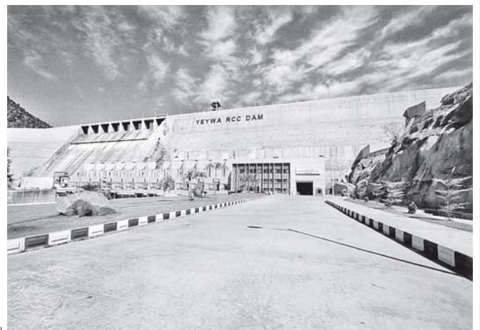
Yeywa Hydropower Plant and RCC Dam.
