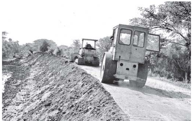
Heavy machinery at work at Thongwakyun embankment road.
