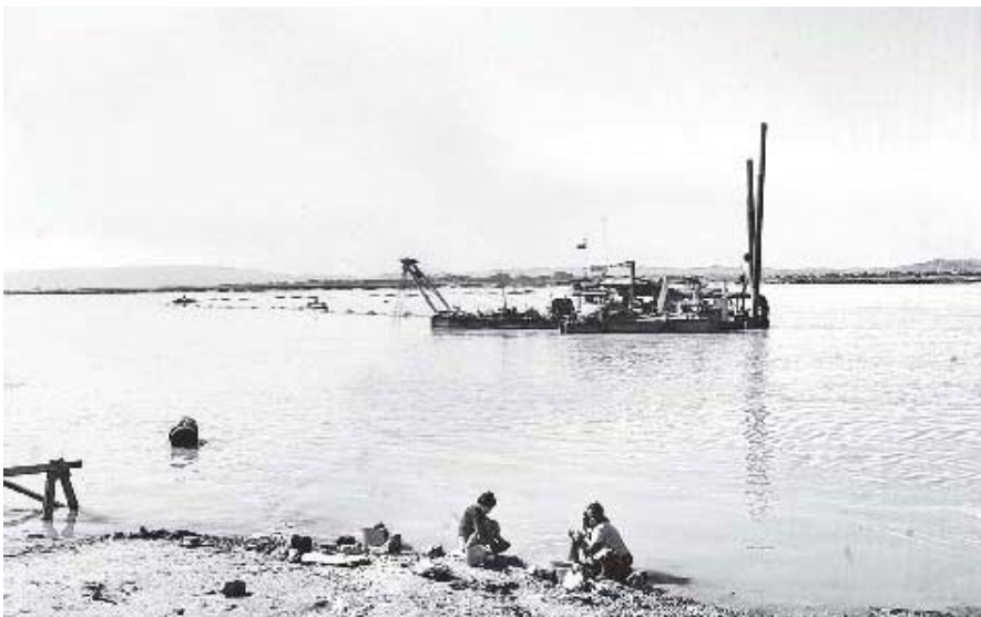
Workers dredging of silt in the water course for safety run of watercrafts at Gawwein Jetty in Mandalay.
