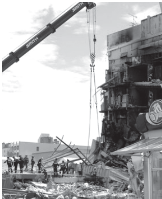
Search and recovery operation personnel work at the destroyed CTV building in Christchurch, New Zealand, 24 Feb, 2011 after the city was hit by a 6.3 magnitude earthquake on 22 Feb. INTERNET
