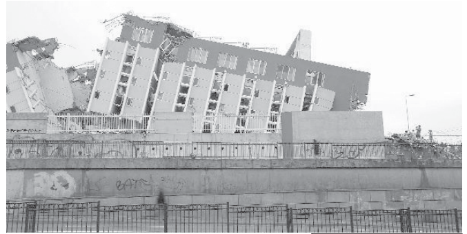
The debris of a house is seen in Concepcion, about 500km south of Santiago, capital of Chile, on 24 Feb, 2011. Concepcion, among the areas hit by a major earthquake and tsunami on 27 Feb, 2010, marks the first anniversary of the 8.8 magnitude earthquake.—XINHUA
