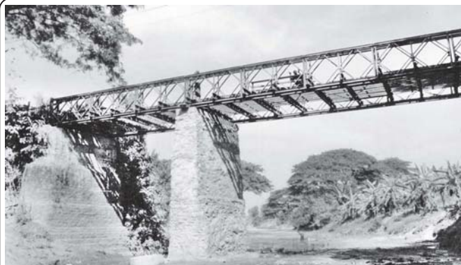
Photo shows Tatkon Creek Bridge at the entrance to Kyunhla.
