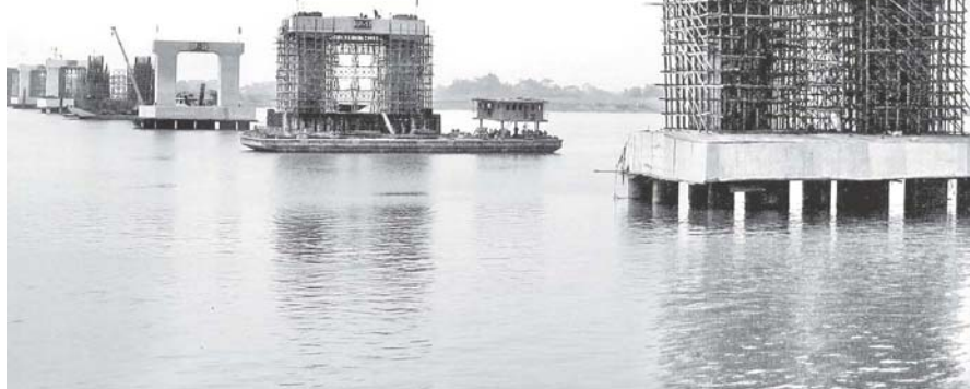
Photo shows piers of Ayeyawady Bridge (Nyaungdon).
