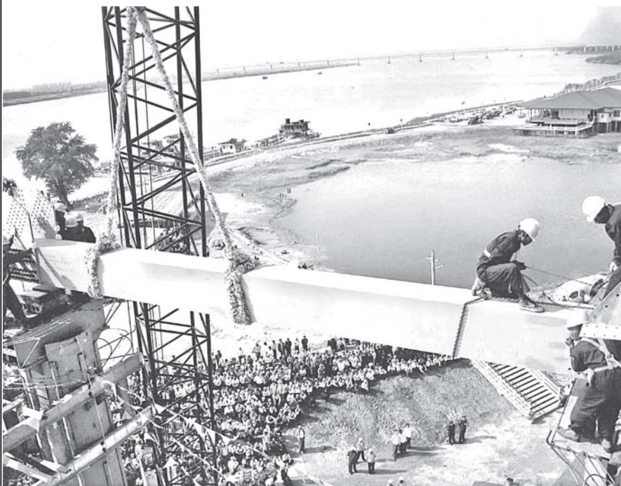
Myanmar engineers install first iron frame at Ayeyawady Bridge (Nyaungdon).
