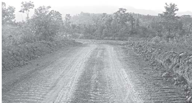
Photo shows progress of Ayechantha-Thitkyitaing Inter-Village Road.
