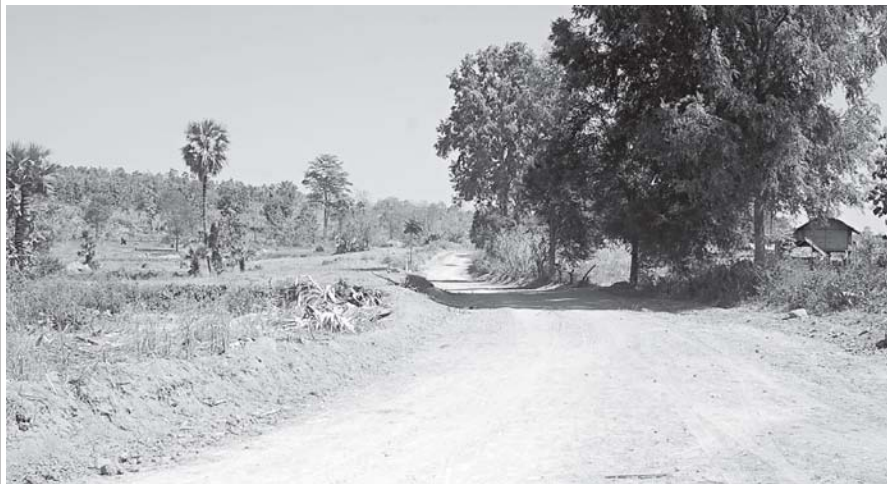
Photo shows progress of Kyetyin-Gaungbwa-Letpan Inter-Village Road.
